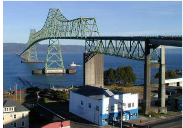
Figure 1 The Astoria-Megler Bridge
